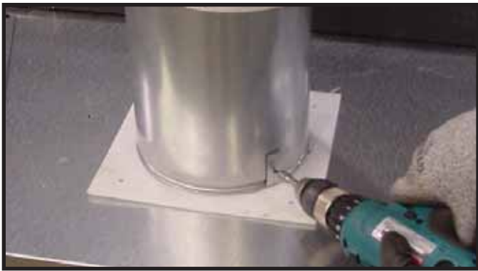
Figure 9.6 To attach the first section of vent pipe, make sure to use the fiberglass gasket in the manual bag to seal between the first vent component and the outer fireplace wrap. Use 2 self tapping screws to secure the gasket to the outer wrap.
